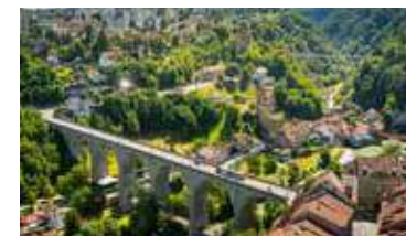
Pont de Zaehringen Zähringerbrücke Zaehringen Bridge (1924)
